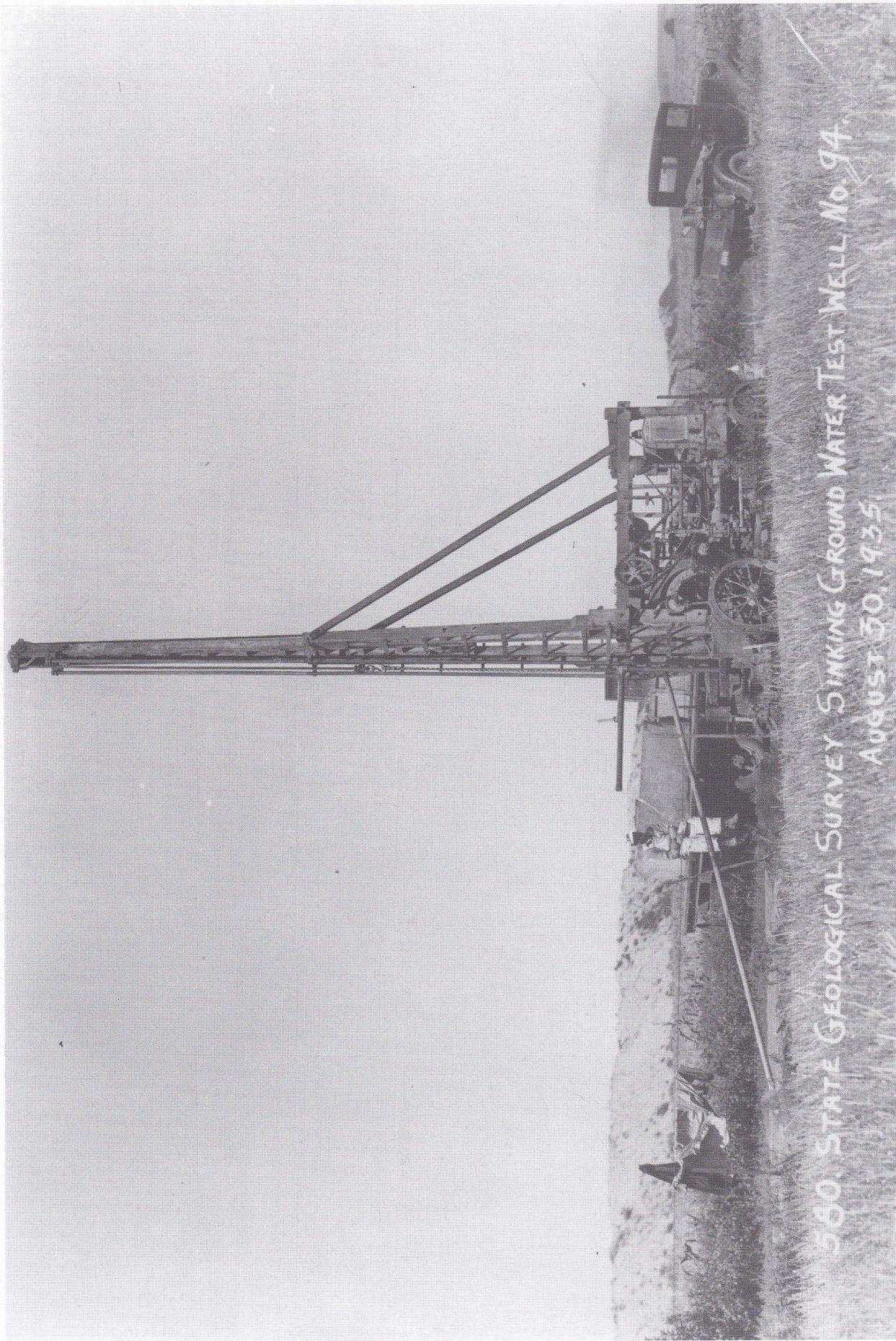
A worker rest a moment as the Conservation and Survey Division (the state geological survey) drills a test hole four miles northwest of Columbus with a Dempster rotary-hydraulic rig near the Loup Power Canal, August 30, 1935. In a state with few outcrops (exposed rock), test drilling is fundamental to understanding the groundwater geology of the state. A cooperative drilling program with the U.S. Geological Survey began in 1930.
